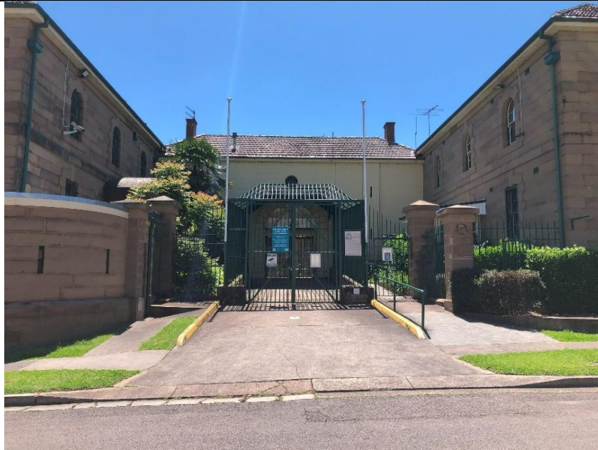
Photo 2 – External view of Main Entry and Gate House
